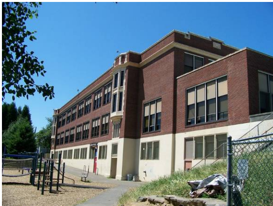
Main building (143A), looking northwest.
