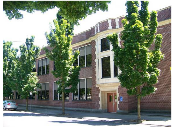
Main building (143A), looking southeast.
