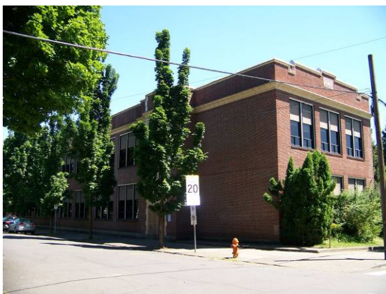
Main building (143A), looking southeast.
